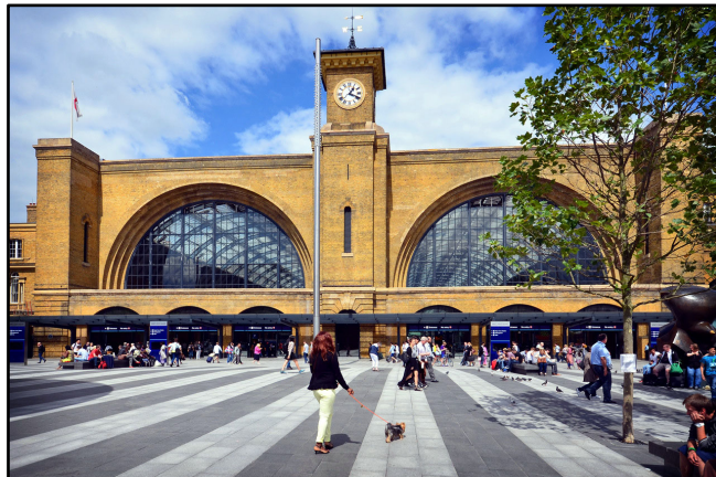
Figura 1 – Telhado da London Kings Cross Station
