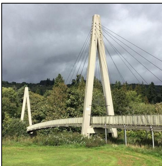
Figura 2 – Passarela Aberfeldy Footbridge
