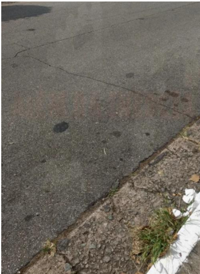
Figura 2. 10 – Trinca Transversal
